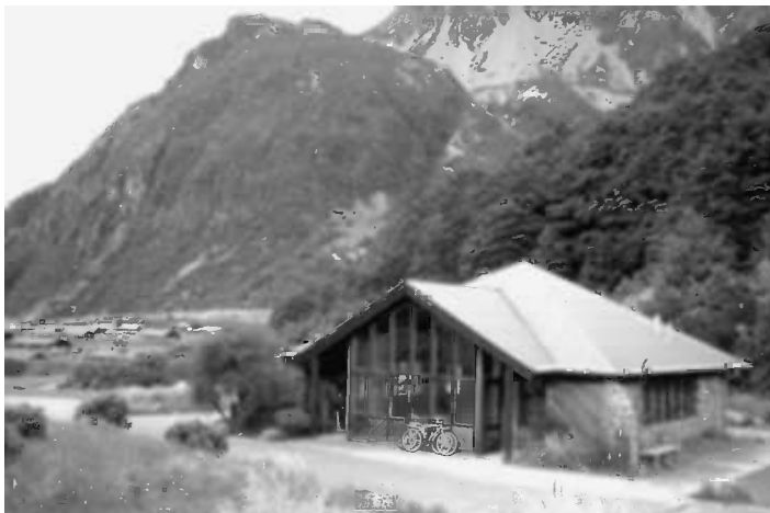
Fig. 8.3. Over time, park managers develop expertise in the design, construction and management of specialized outdoor recreation facilities. The heavy rains and winds of the New Zealand southern mountains require special facilities for the visitors. This shelter in Mt Cook National Park provides shelter for visitors. Shelter in Mt Cook National Park, New Zealand. (Photographed by Paul F.J. Eagles.)
