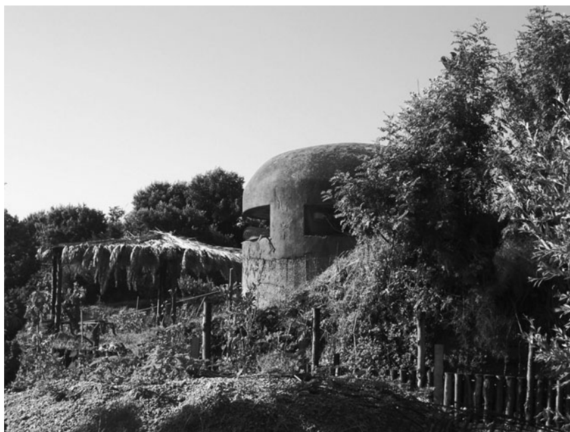
Fig. 6.3. Changing symbols: a Second World War bunker now used as a storage space by farmers (photo: Giovanni Lombardi).
