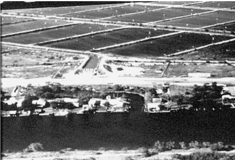
Fig. 15.4. Water intake system at AAA.
