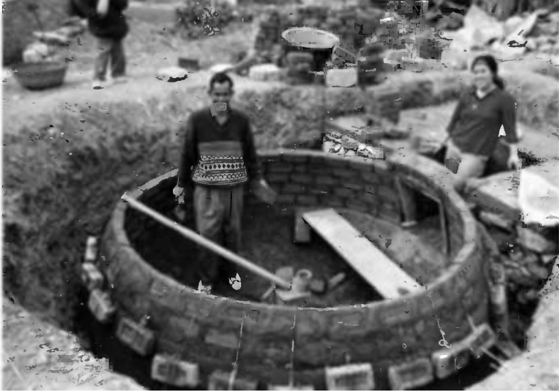
Fig. 14.4. Volunteers preparing infrastructure for installing a biogas plant in Kanda.
