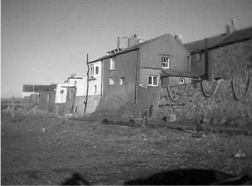
Fig. 6.1. Seafront houses, Ravenglass, Lake District, Cumbria, UK (photograph courtesy of C. Cater).
