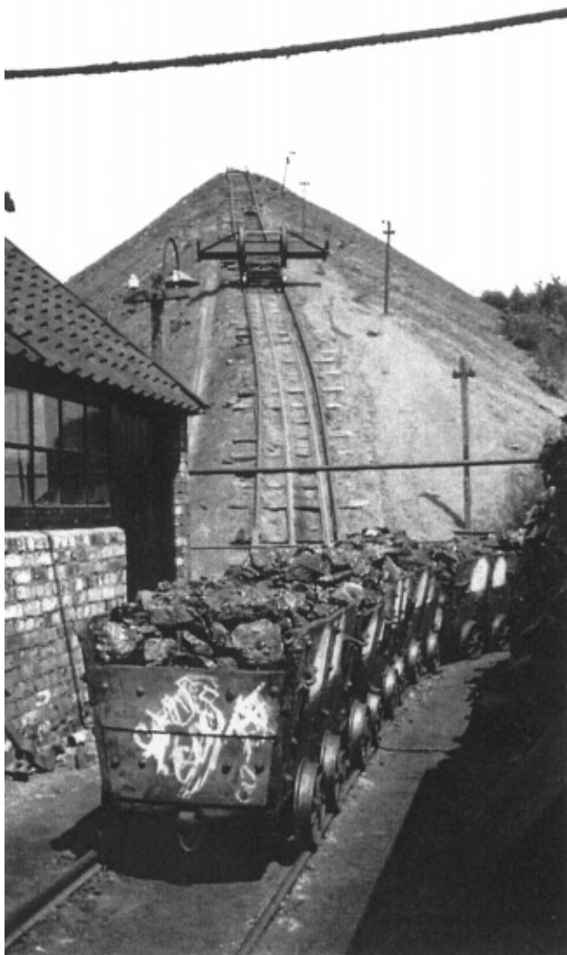
Fig. 10.2. Photograph of the new pit batch, possibly 1930s, showing a Mclean Tipper, the steeper tip form, and the bare condition of the tips when working.
