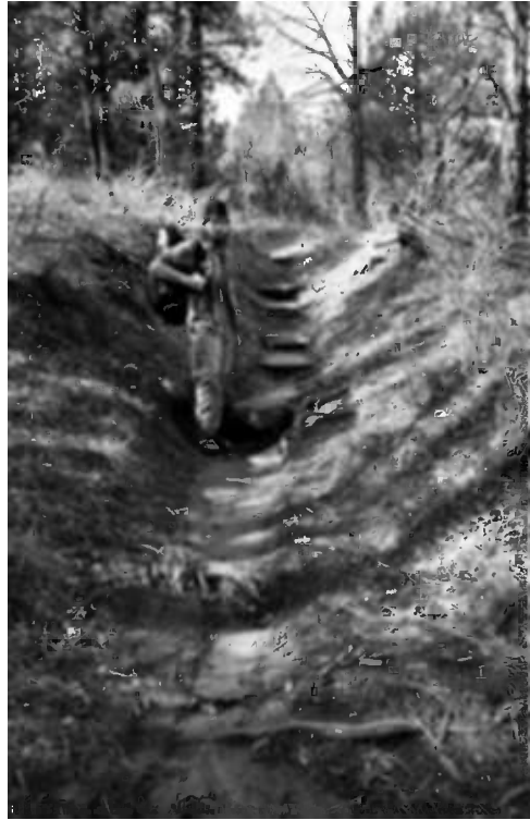
Fig. 13.2. It is impossible to drain water out of this entrenched trail in Zion National Park, USA, due to its low slope alignment angle. Re-routings is recommended to avoid the need for extensive tread work involving erosion control measures and steps on the existing alignment.
