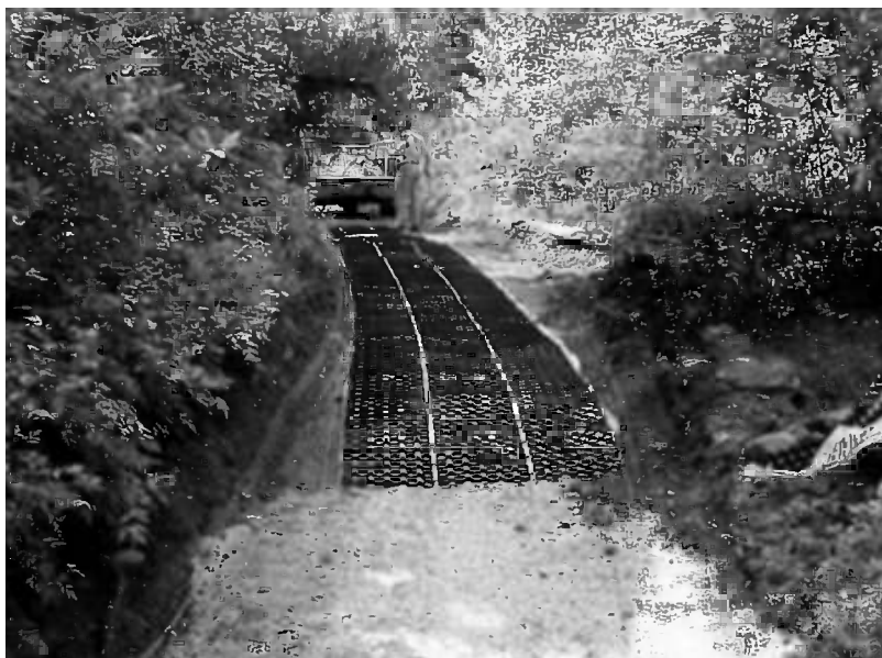
Fig. 13.5. Geosynthetics are applied on this trail in the Daniel Boone National Forest, USA, to improve trafficability for all-terrain vehicles and horses.
